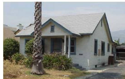
Before compressed air foam
